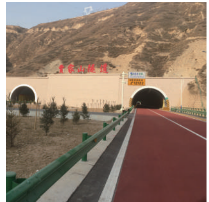
Lanzhou Highway Tunnel, China
