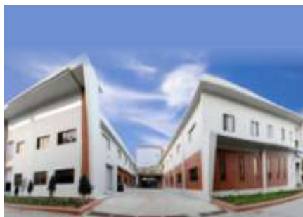
Tempsens Instruments U# II Cable Plant
