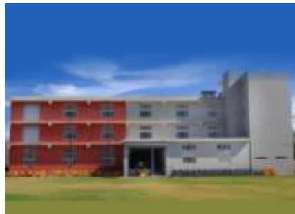
Tempsens Instruments U# IV Cable Plant
